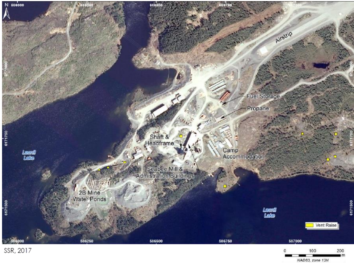
Figure 18.2 Seabee Gold Operation Mill Site Infrastructure
