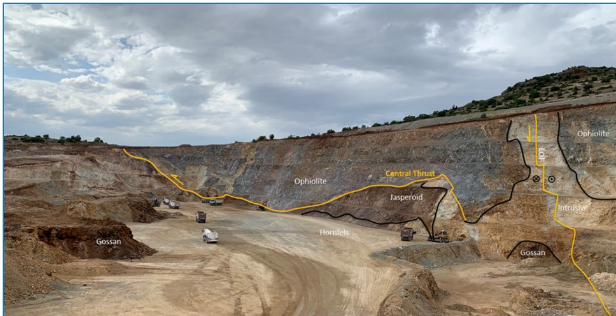
Figure 6.9 Geological Mapping within Çakmaktepe Central Pit
